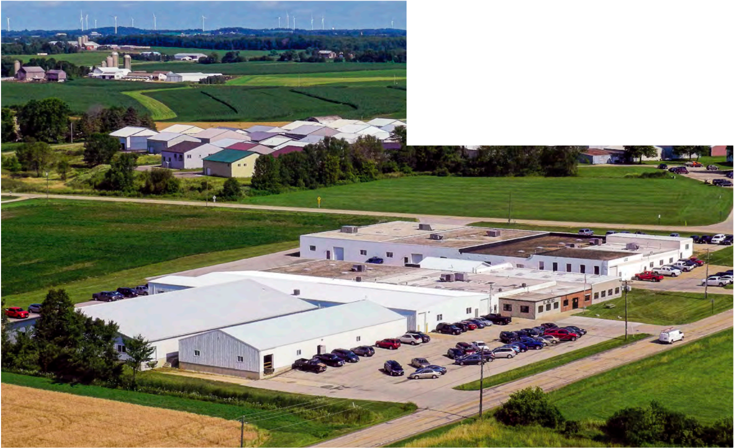
OUR PRODUCTION FACILITIES IN HARTFORD, WISCONSIN
